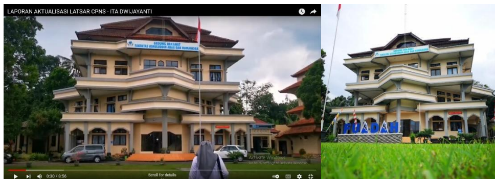
Figure 10. Exterior Images Before and After Construction of Identity Signage
